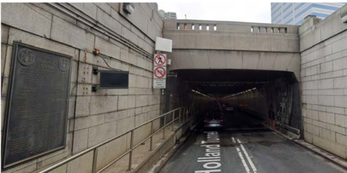
Figure 5 Entrance to Holland tunnel, Jersey City NJ
