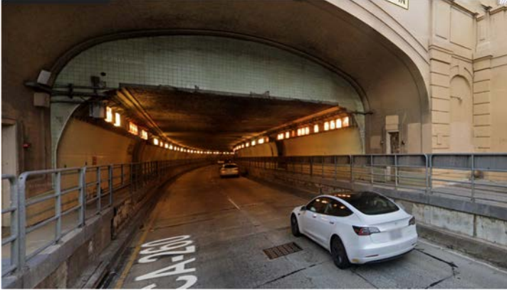
Figure 6 Raised walkways for pedestrians, Posey tunnel, Oakland CA
