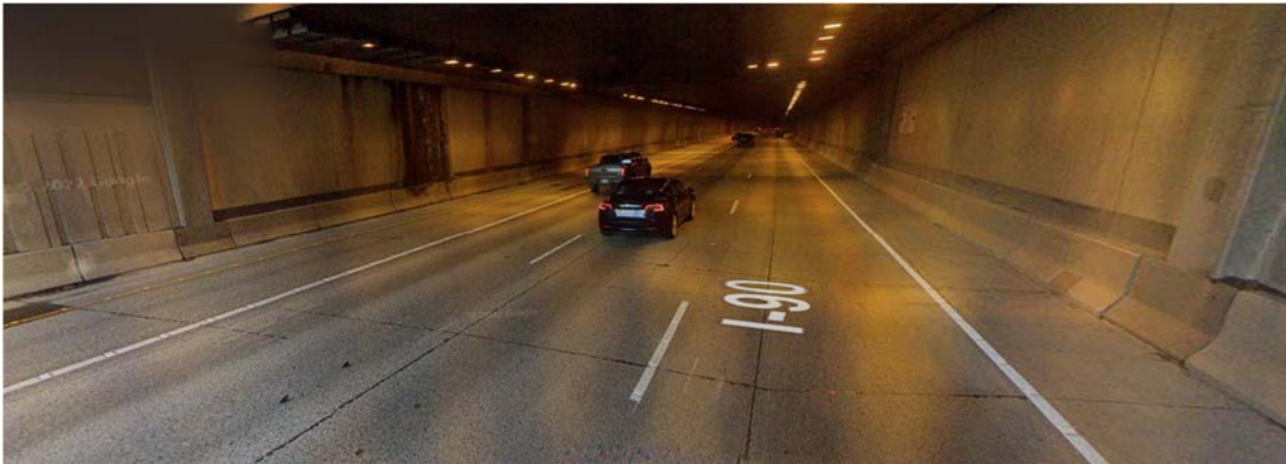
Figure 8 Tunnel with shoulders, no walkways, I-90 Mercer Island, WA
